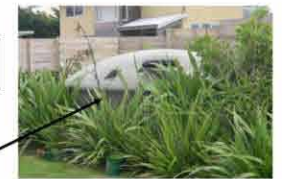
Rainwater collection tanks
