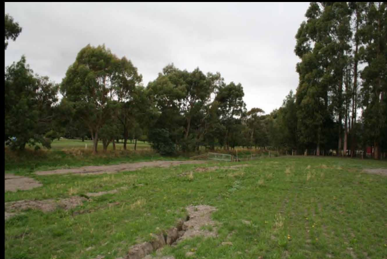
Halswell River levees ripped after the February earthquake
